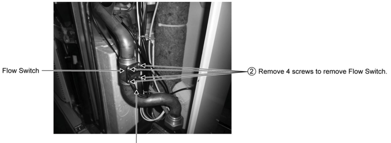
① Disconnect the connector of CN-FLOW (YLW) from the Electronic Controller Board.
